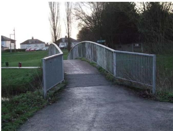
Milton Keynes: typical overbridge design on shared use Redways. Note that the thickness of the parapet wall provides additional protection that obviates the need for a higher parapet.
