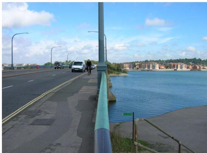
Bristol: signed cycle route on bridge over M32. Parapet height 1.1m
