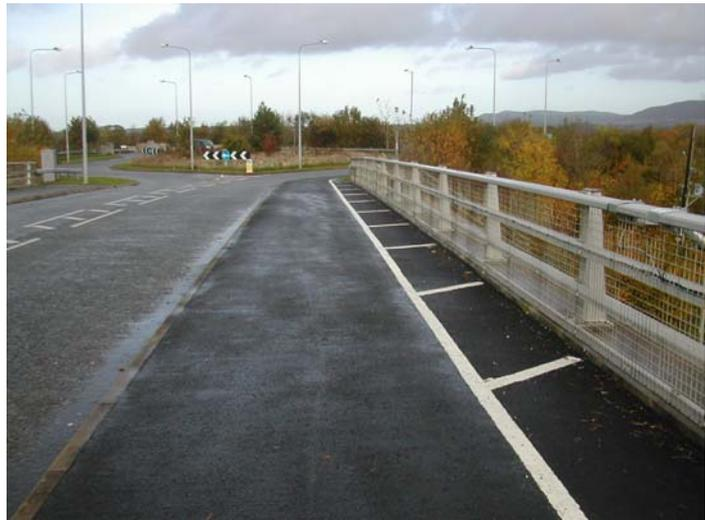
Bothwell Bridge over the A725 dual carriageway north of Hamilton. The parapet height is 1.1m and white lines have been used to pull the cyclists away from the parapet edge and so the safety auditors deemed no parapet works were necessary. The route is an unsegregated shared use section of path on NCN 74.
