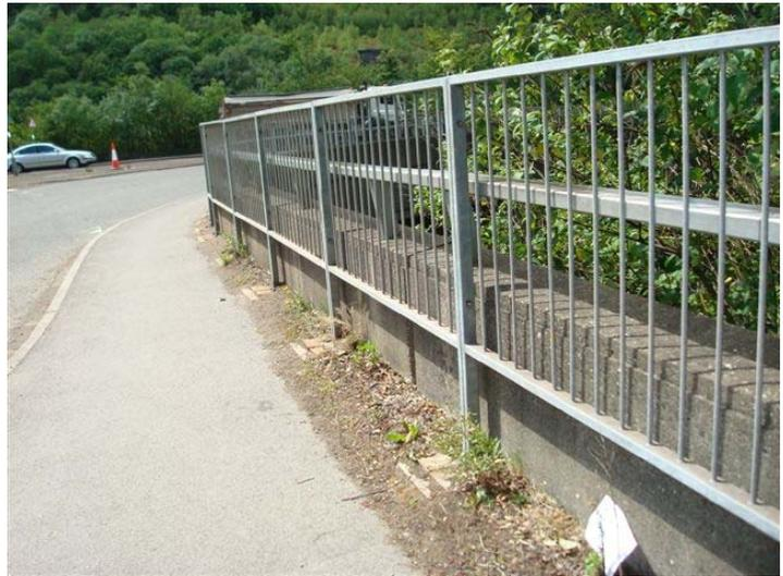
Havering: raised pedestrian guard railing - undertaken because the council felt that there was a significant drop from the edge of the path into an adjacent watercourse.
