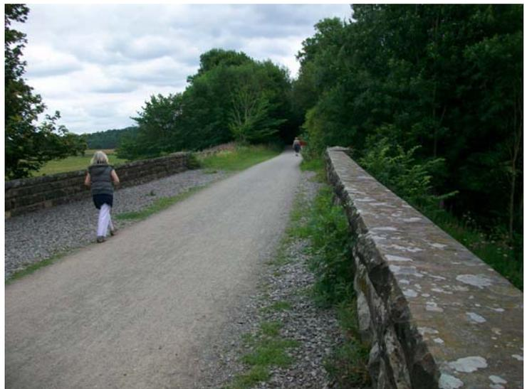
Bristol: whilst not a bridge, the 'Chocolate Path' alongside River Avon has a 970mm parapet height.
