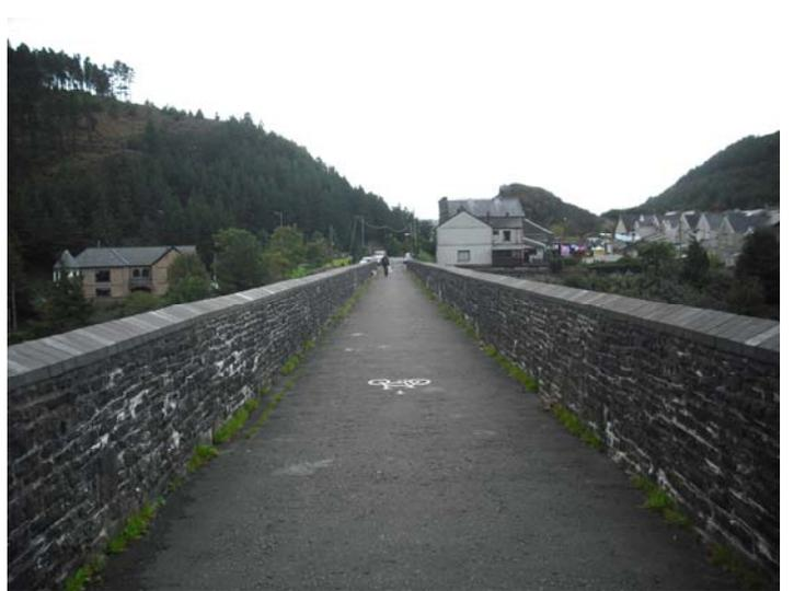
Monsal Trail, height is approx 1m and the bridge passes over highway. The path alignment keeps users away from the parapets and the thickness of the parapet wall provides additional protection
