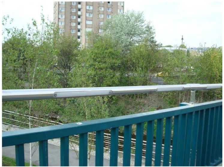
Taff Trail over a trunk road near Taffs Well: pedestrian guardrailing installed in front of existing parapet.
