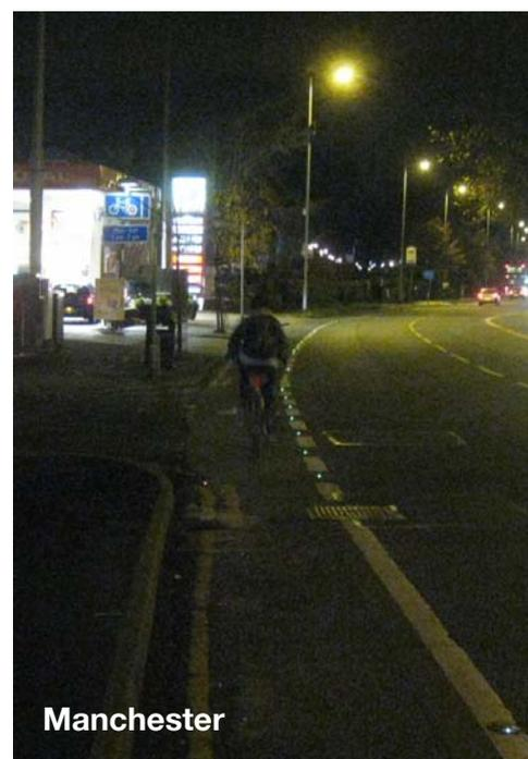
are spaced at between 8 - 10 metre intervals along the cycle lanes depending on the straightness of the road (8 metres on sections with bends and 10 metres on straight sections). Green studs are spaced at 2 metres intervals across side road junctions / lay-bys and busy entrances / exits.
