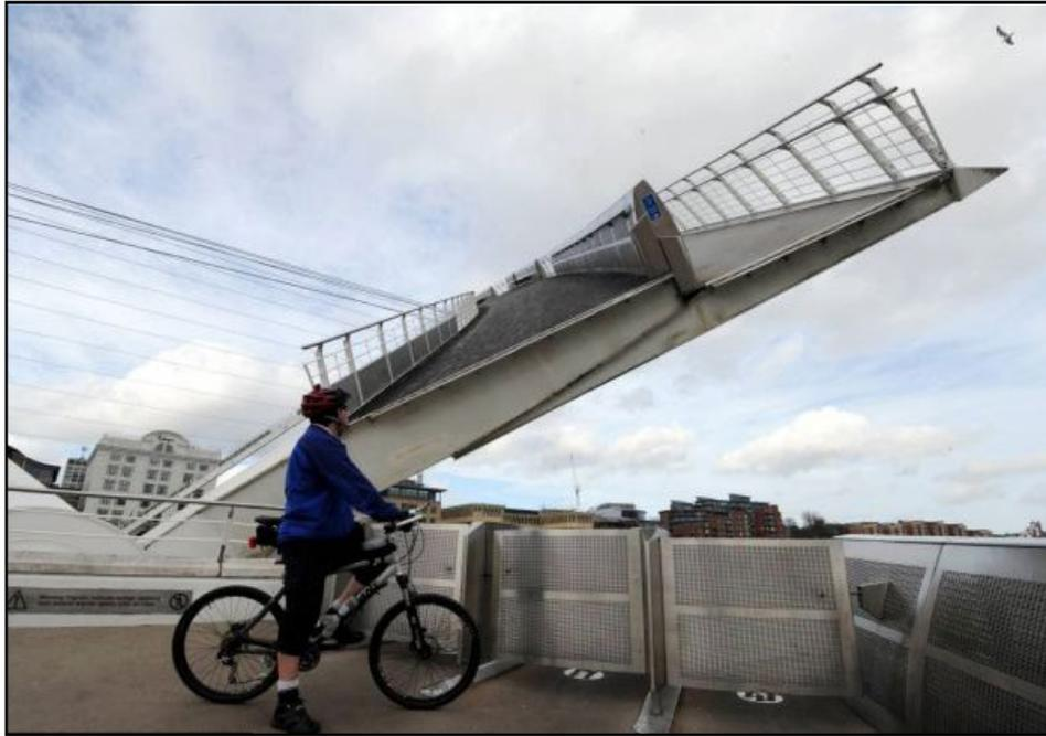
Figure 3: Cycle and pedestrian barriers at the Gateshead Millennium Bridge<sup>2</sup>
