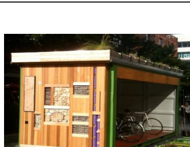
Green roof and timber cycle shelter.
