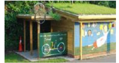
Green roof bike shelter by the Grass Roof Company.
