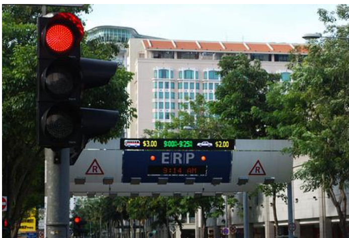
Singapore ERP charging gantry, Creative Commons Image
