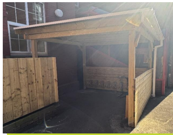
Figure 1: New bike shelter at Holton Primary School. ©Holton Primary School
