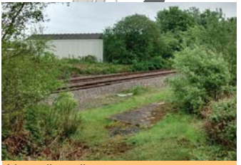
Live railway line
