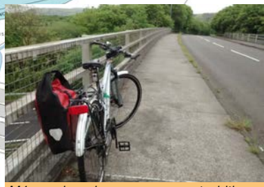
M4 crossing – increase pavement width to provide shared use path and increase parapet height to 1.4m
