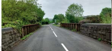
M4 crossing – increase pavement width to provide shared use path and increase parapet height to 1.4m
