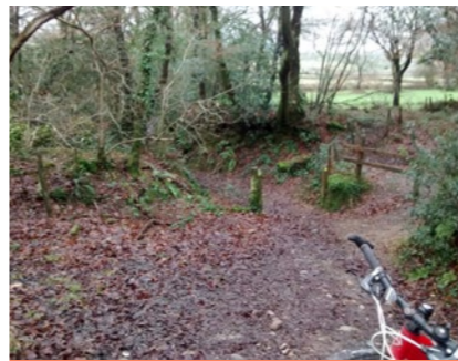
Up-grade surface that is suitable for all users (walk, cycle, horse), Look at options to increase usable width and surfaces that can reduce maintenance
