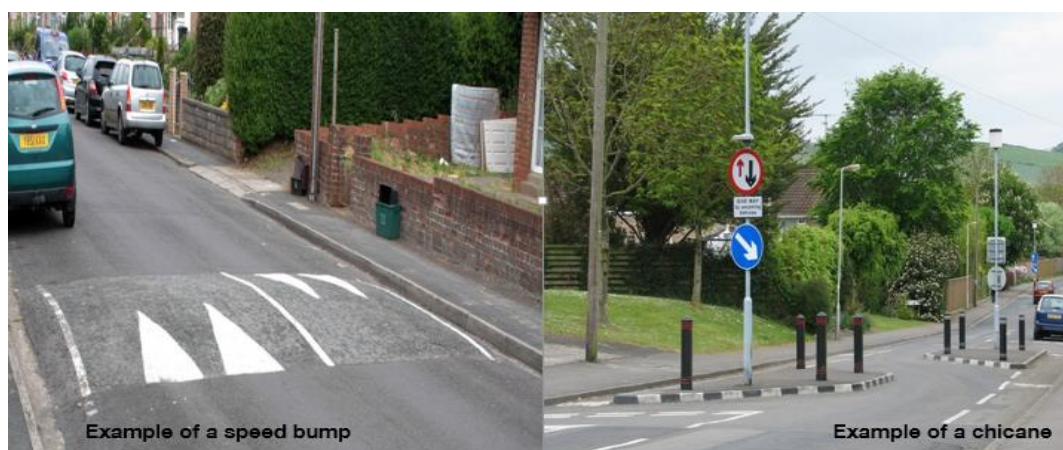
Figure 2: Example of physical measures
