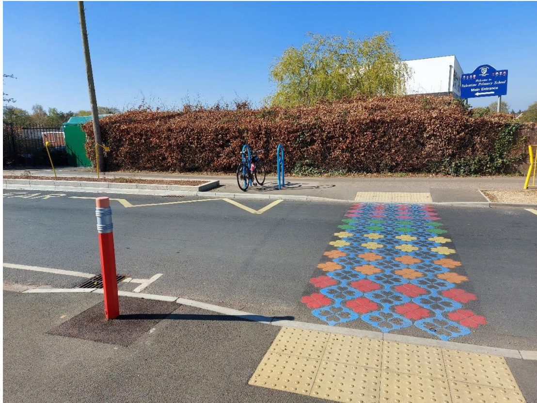
Figure 11: Thermoplastic art added to Valentine Avenue outside Valentine School in Southampton.
