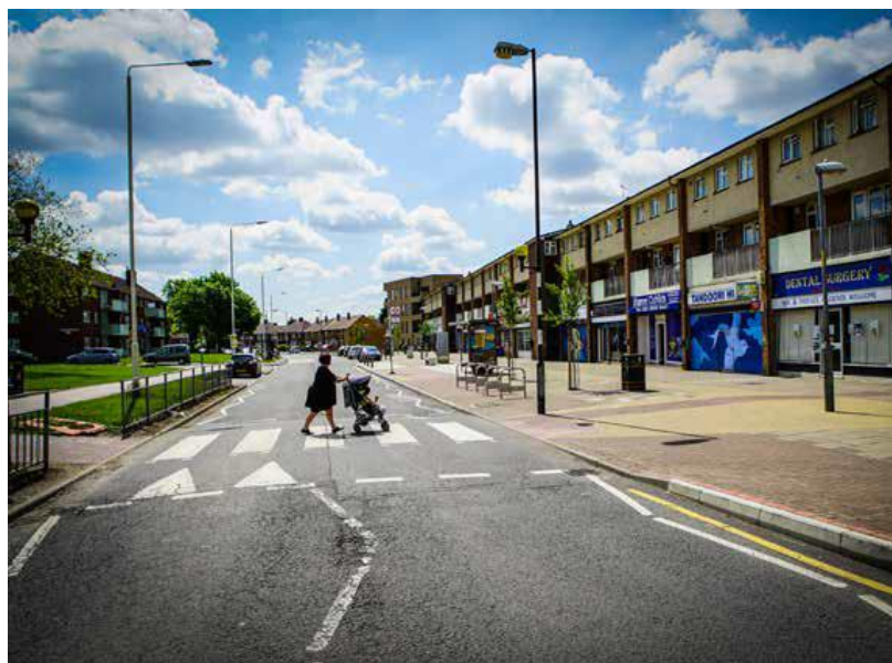
Figure 11: Improved crossing points and resurfaced pavements
