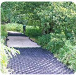
An above-ground no-dig construction method will be used to protect existing trees. Image source: Geosyn.co.uk
