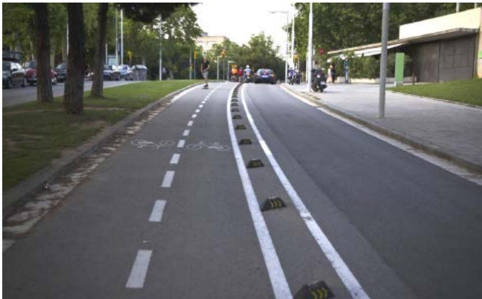
Example of a semi segregated cycle lane (Picture courtesy of Transport for London) in which armadillos are placed between mandatory cycle lane markings. In the case of Meadow Place Road the cycle lane would be unidirectional.
