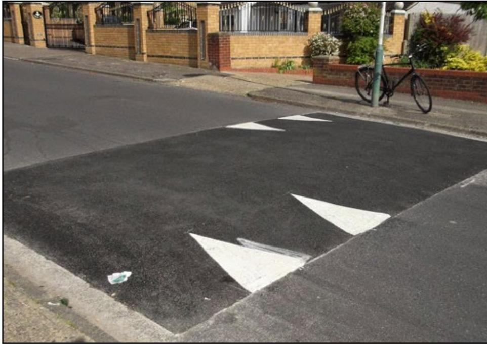
Figure 7: Sinusoidal speed hump
