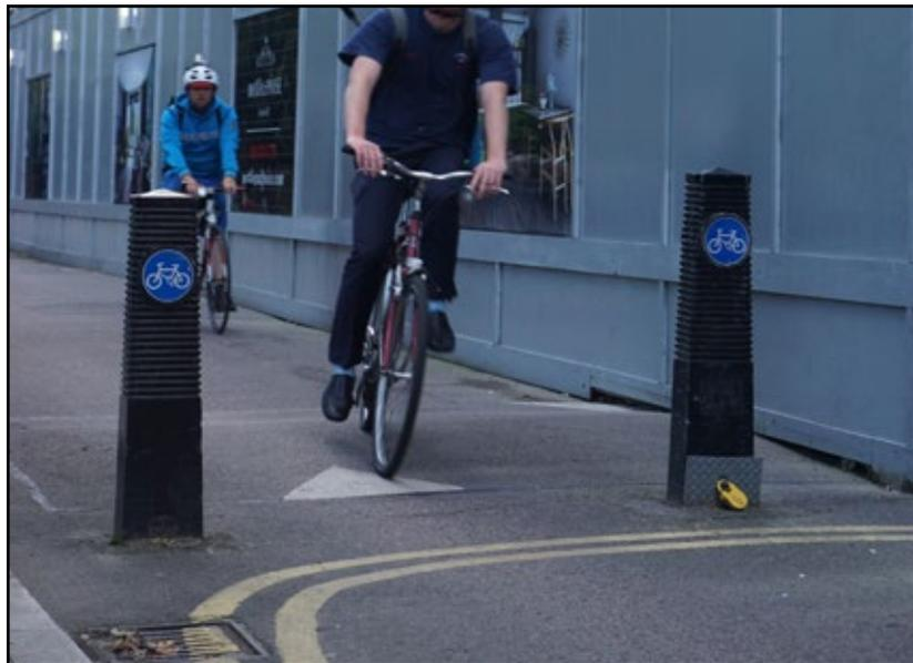
Figure 8: Example of de-mountable bollard, on right
