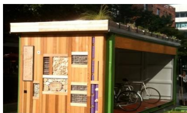
Green roof and timber cycle shelter.
