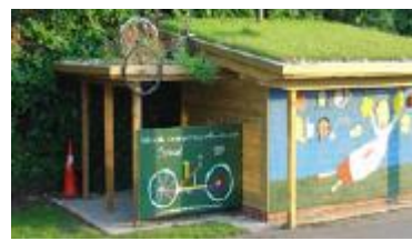
Green roof bike shelter by the Grass Roof Company.
