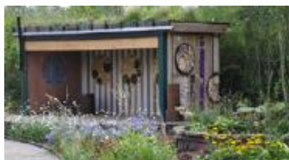
A recycled shipping container turned into a habitat shelter.
