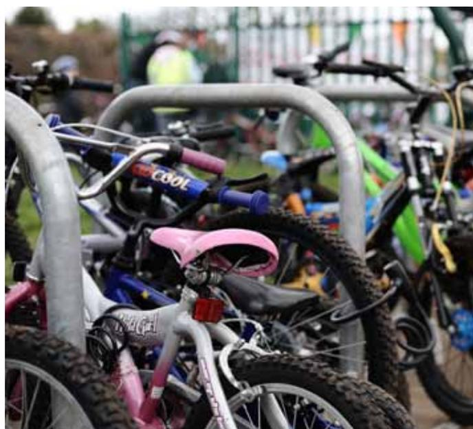
**Sheffield stands** (above right) can be fitted singly or in toast racks. They are robust, low maintenance and easy to fit. You can fit two bikes to each, which can be locked by both frame and wheel.
