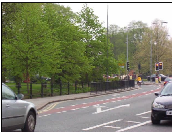
Cycle lane on the off side of a filter lane, Cambridge
