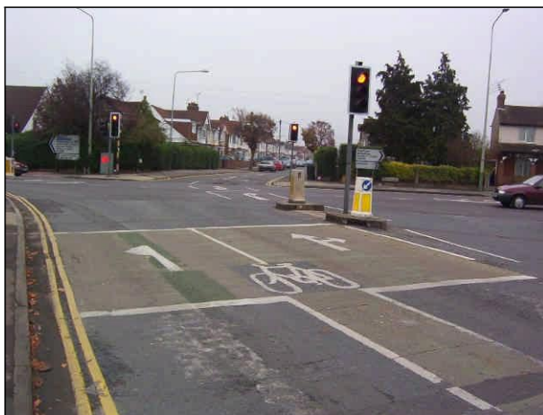
ASL at signals with filter, Swindon
