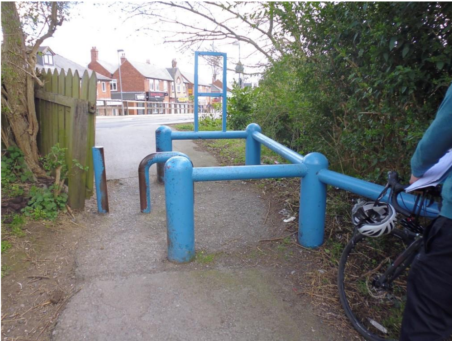
Figure 4 – A barrier on the Foss Islands path before changes were made (c) 2016 Sustrans
