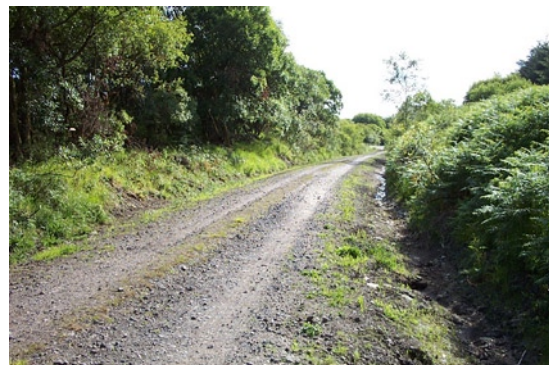
Forest road with good side ditch
