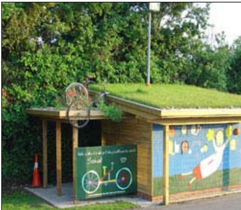
Green roof bike shelter by The Grass Roof Company
