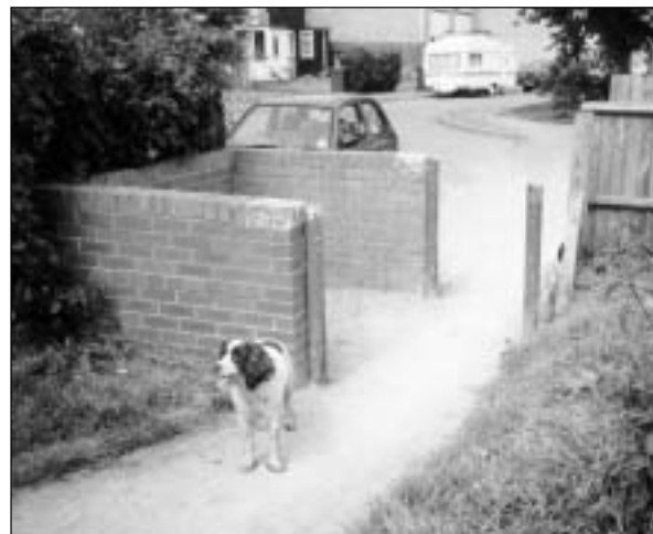
Central barrier removed leaving a gap.
