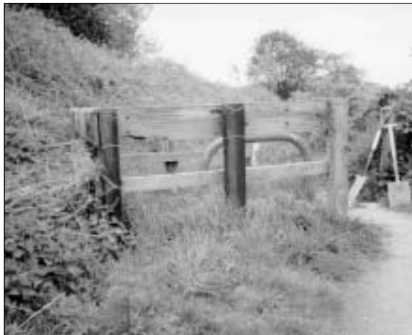
Restrictive access control
