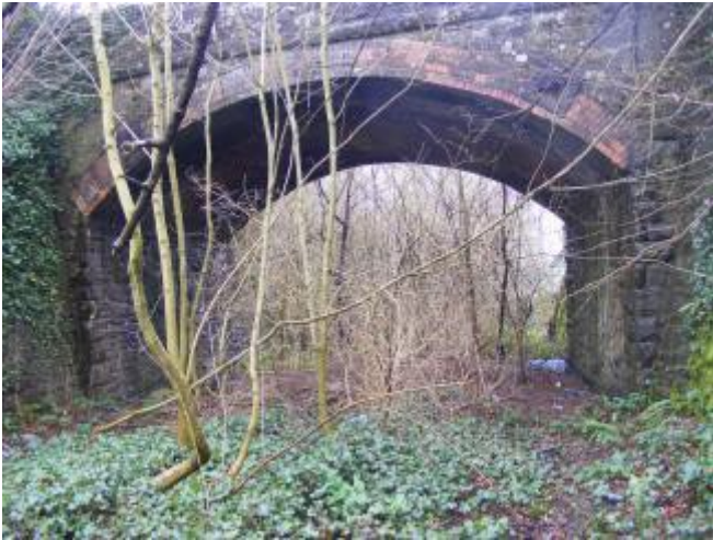
Figure 31. Bridge at start of Section 3, looking east
