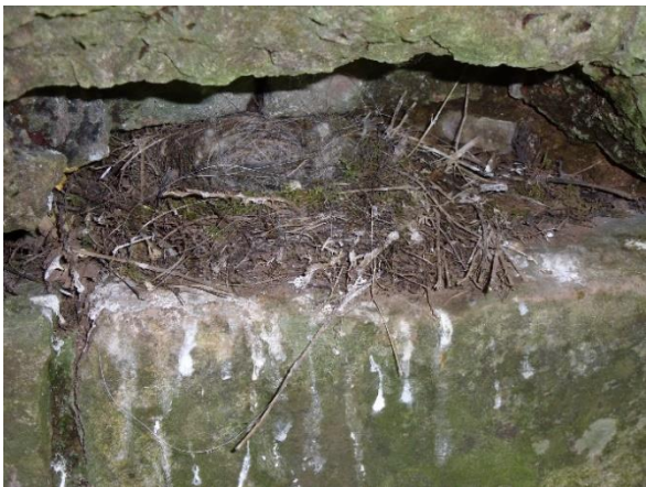
Figure 4 Birds' nest under bridge over Berthin Brook (target note 2)
