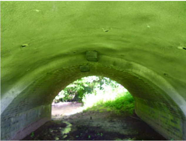
Figure 10 Bat bricks under Berthin Bridge (target note 21)
