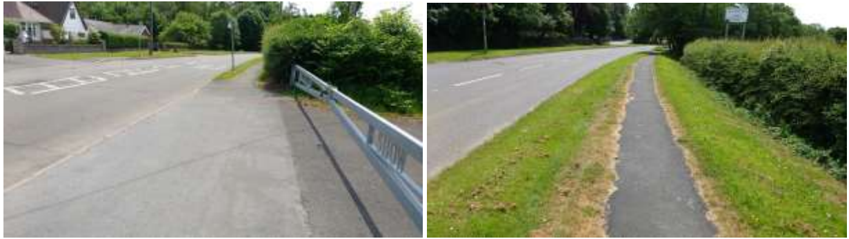
Photo's 3.15 and 3.16 – Pentre Road and the existing footway.
