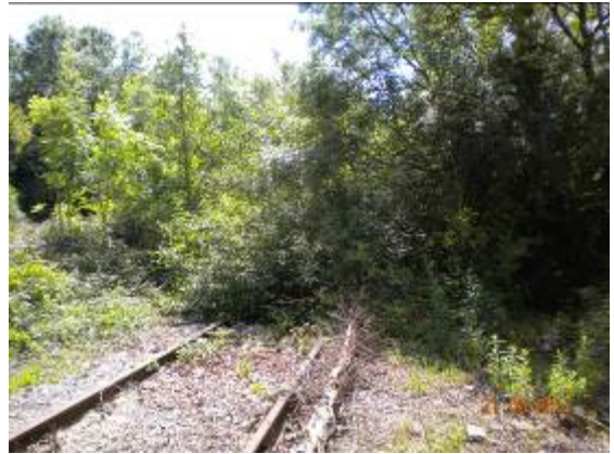
Track partly blocked by scrub
