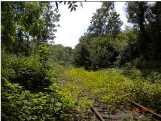
Track section north of bridge, facing south
