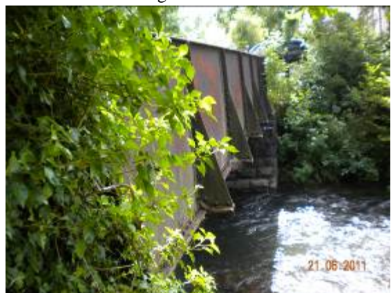
Metal bridge with stone supports
