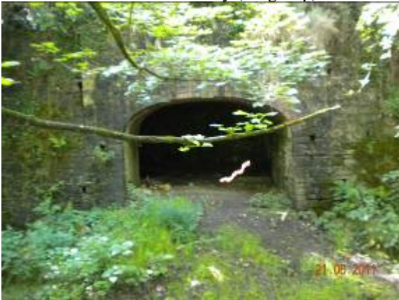
Tunnel & overbridge, old Brynmenyn colliery
