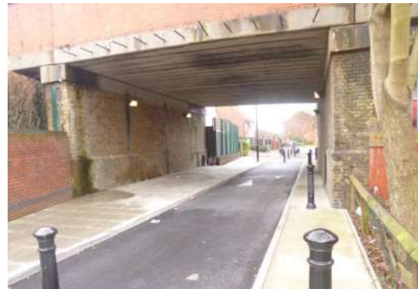
Images: Stevenson Crescent before (above) and after (below)
