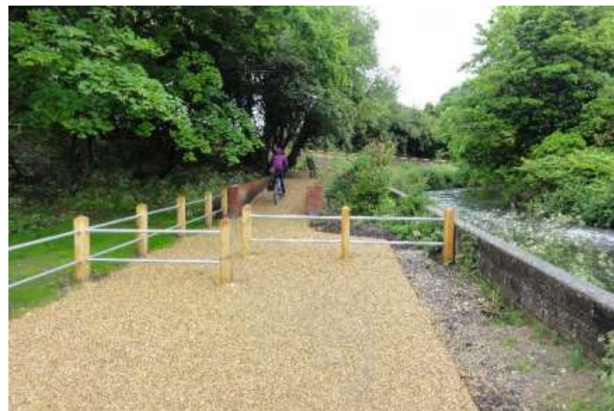
Image: Wide access controls at the Wandle Trail enable conflict free journeys for cyclists and pedestrians along a traffic-free greenway
